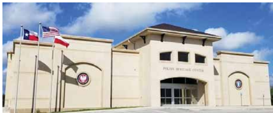
PHC building facade
